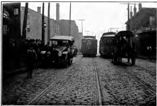
WHERE A DOUBLE TRACK OVERBURDENS A NARROW STREET On this street tire trouble held up seven cars for fifteen minutes. Owners of property stated that they had difficulty in getting coal companies to deliver coal, owing to the tie-up to traffic which the delivery necessitated.
